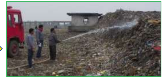
Sprinkling of water for compressing the heap
