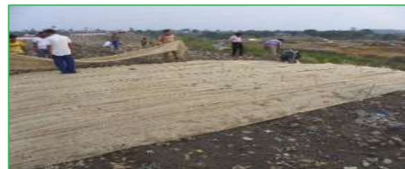
Covering of surface with Jute & other capping Material
