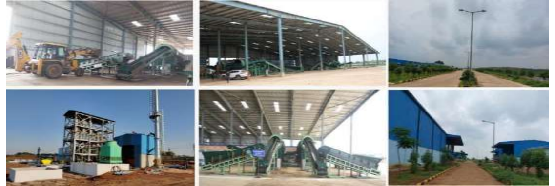
Sakri Integrated Solid Waste management Facility (Raipur)
