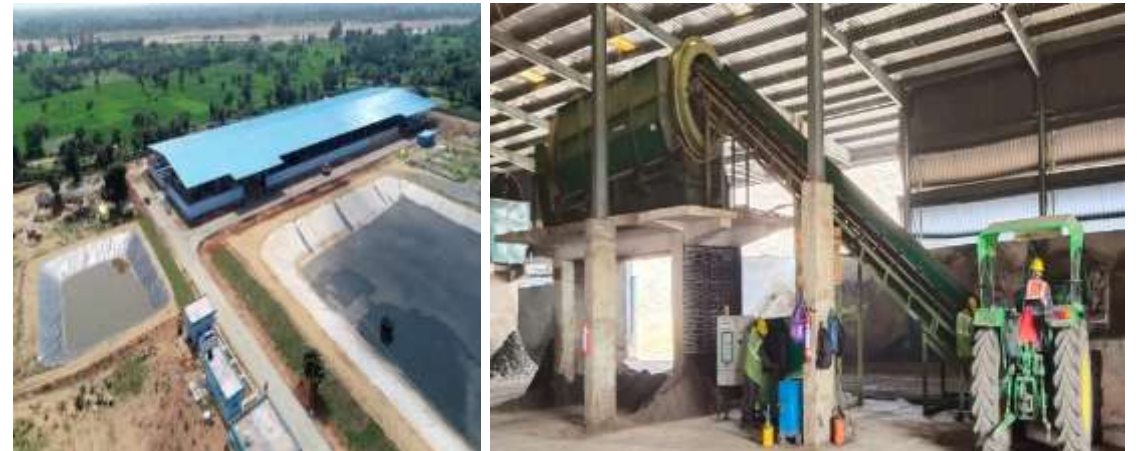
Kachhar Integrated Solid Waste management Facility (Bilaspur)
