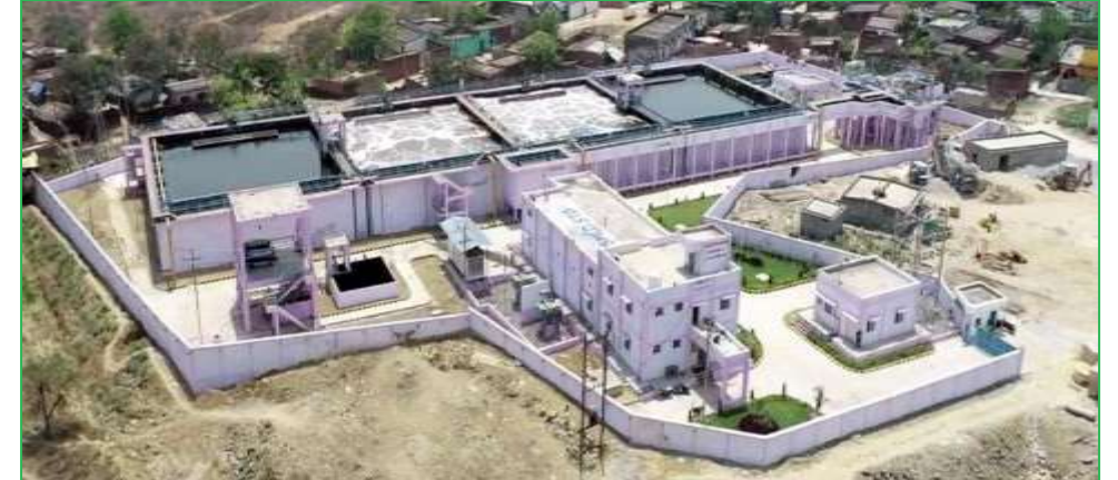
Raigarh (Banjipali): 25 MLD
